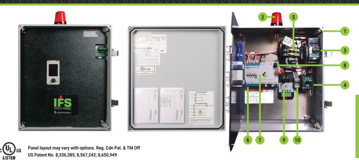
The Next Generation IFS simplex control panel utilizes an innovative circuit board design enclosed in a touch-safe housing to control one 208/240/480 and 600 VAC three phase pump in water and sewage applications. These newly redesigned IFS panels feature an easy-to use color LCD interface located on the inner door for programming and system monitoring. The panel configuration can be easily converted in the field to either a timed dose or demand dose through the LCD interface.
