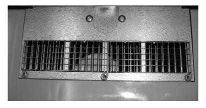
6. Reinstall the three (3) Philips-head screws to secure the heatsink cover to the drive.
