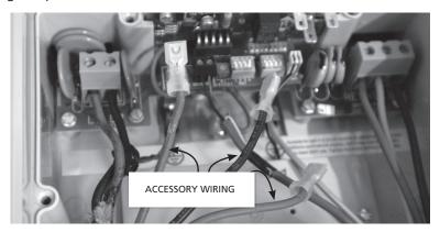
6. Attach wires to NO, NC and COM as needed.
